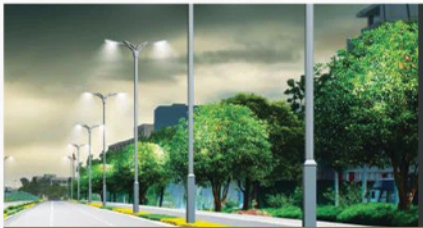
Electric Poles with Street Lighting
